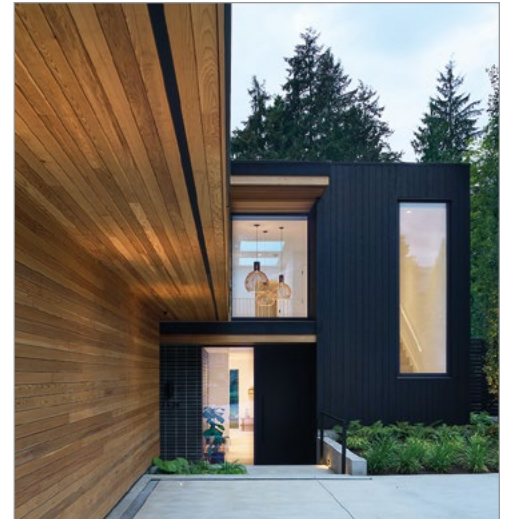
The strategic interplay of contrasting color at Bluebonnet is easy to achieve because western red cedar is pitch and resin free, which means it accepts and holds finishes beautifully. Bluebonnet. Architect: Shelter Residential Design. Photography: Sama Jim Canzian.
