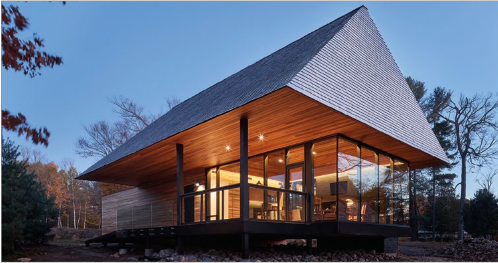
The choice of an exterior wood finish for western red cedar depends upon the desired appearance and the degree of protection required. Bigwin Island Club Cabins. Architect: MacKay-Lyons Sweetapple Architects. Photography: Doublespace Photography.
