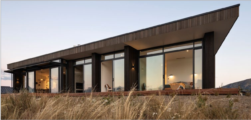
Charcoal noir is a very popular look for siding and was traditionally done by charring the wood, a technique used in Japan called Shou Sugi Ban. Ruby Ridge House. Architect: Condon Scott Architects. Photography: Simon Devitt.
