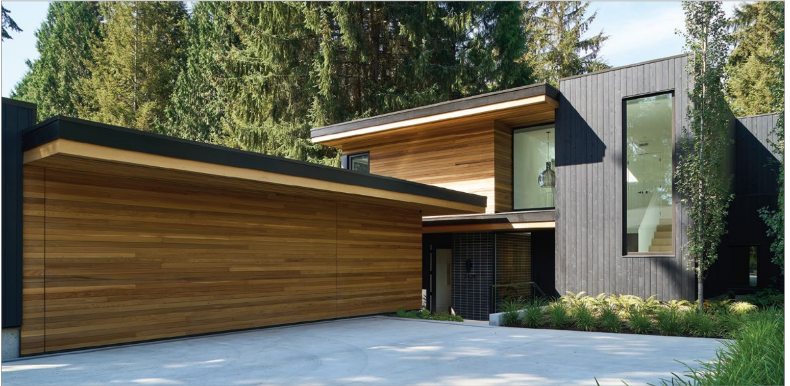
Black and natural siding finishes create a striking contrast in natural settings. Bluebonnet. Architect: Shelter Residential Design. Photography: Sama Jim Canzian.
