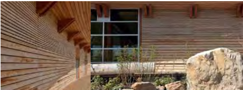
Cedar Cladding Detail Base of Wall
