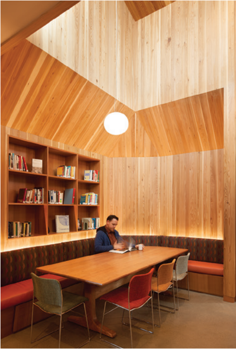
Inside the Unitarian Universalist Fellowship of Central Oregon, a majority of the interior walls are finished in clear Western Red Cedar T&G siding in two custom profile shapes to create warm, inviting, and extremely humane spaces. Unitarian Universalist Fellowship of Central Oregon by Hacker. Photo by Lara Swimmer.
