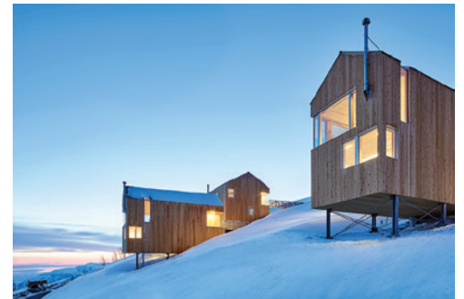
To help minimize the project's overall footprint, MacKay-Lyons specified naturally beautiful Western Red Cedar for the shingled roofs, the vertical cedar wall cladding, and the soffits. Horizon Neighborhood by MacKay-Lyons Sweetapple Architects. Photo by Doublespace Photography and Paul Bundy
