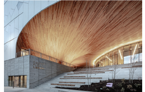
Each cedar panel curves down toward the ground, creating an entrance intended to attract the public into the building. Calgary Central Library by Snøhetta & DIALOG. Soffit by StructureCraft. Photo by Lucus Epp & Julian Parkinson.
