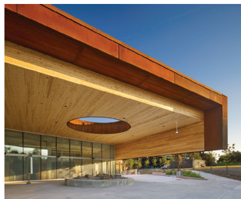
The Perkins + Will team ensured a welcoming vibe through the inclusion of a warm, expansive, 20m cantilevered overhang at the main entrance. The soffit of this key entryway feature is a knotty grade of naturally beautiful Western Red Cedar. Kawartha Trades and Technology Centre by Perkins + Will. Photo by Tom Arban and Scott Norsworthy.
