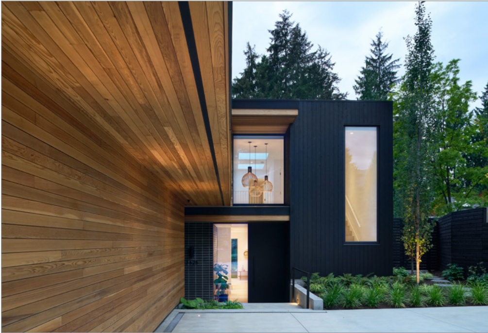
Western red cedar soffits can be used to coordinate with exterior cedar siding or create a seamless aesthetic with interior cedar ceilings. Design by Shelter Residential Design. Photo courtesy of Sam Jim Canzia.
