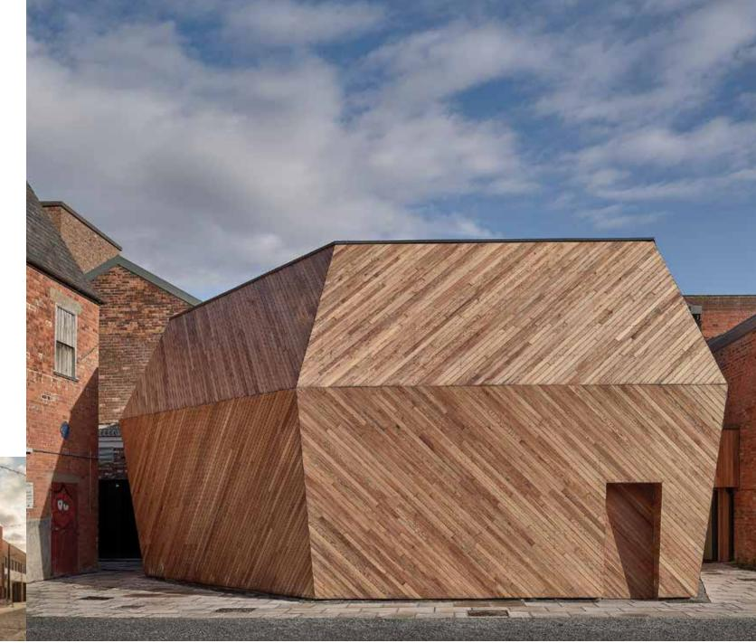
Acoustic performance was a primary concern, as the expanded venue needed to prevent sound transfer to the surrounding new developments. A super-insulated timber frame structure, clad entirely in Western Red Cedar, enhances both thermal efficiency and soundproofing.
