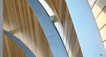
The roof shells were prefabricated off-site, then transported by truck, lifted into place by crane and secured to steel pin connectors cast into the concrete slab. Once installed, the shells were connected with plywood splice plates, and the cedar lining installed.
