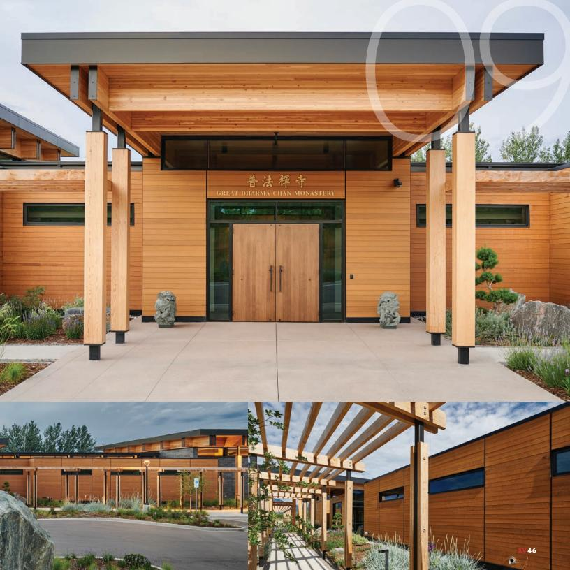
and exposed Cross-laminated timber (CLT) roof panels for this 21,000 square foot meditation hall. It's a choice that offers a minimal carbon footprint and a beautiful aesthetic.
