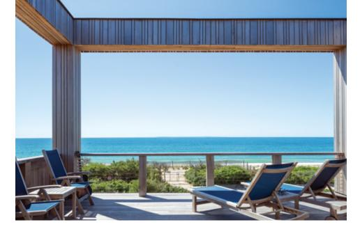
"A high priority was placed on the selection of long lasting, durable materials and development of construction details to withstand the severe weather," explains Albert Garcia, AIA, KITE Architects' Principal. "As such, the house is clad with a rainscreen wall system comprised of Western Red Cedar arranged in a pattern that follows a rigorous and consistent module as it cascades across projections and recesses."
