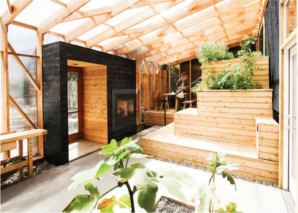
Unique treatments not typically achieved using standard factory finishing treatments include sand blasting, wire brushing, blasting with walnut shells, hammering or beating the wood with other tools, and charring the wood with a blow torch to achieve the Shou-Sugi-Ban look, as seen here on the entryway.
