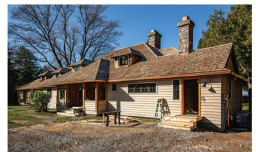
The exterior walls are clad with with engineered, knotty 3/4" x 8" beveled Western Red Cedar siding from British Columbia.
