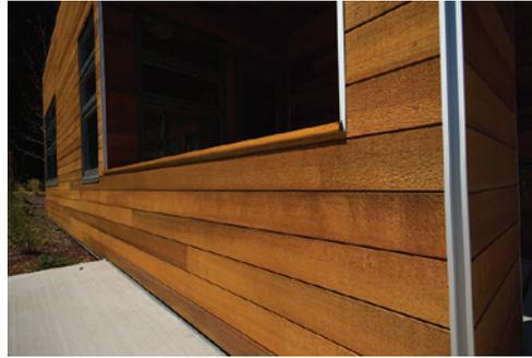
or Tex grade bevel siding is recommended for use as sidewall covering where the distinctive charm of a rustic saw textured appearance is desired. This grade allows limited characteristics that do not detract from serviceability.<sup>11</sup>
